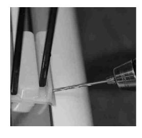
Step 32: Adjusting the Anti-Jump Screws: EASCO Bi-Pass Shower Doors are equipped with an Anti-Jump Feature. When properly adjusted the Anti-Jump Screw will not allow the roller to jump from its track. Once the doors are aligned and the center-guide is installed we can set the Anti-Jump Screw.
