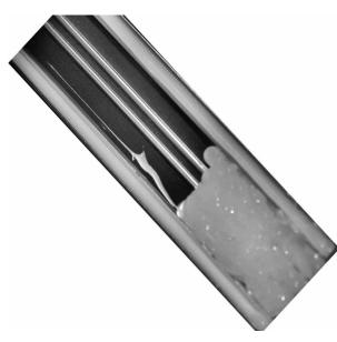
Step 10: Apply a continuous bead of Silicon Sealant in the 2 channels on the bottom side of the Bottom Track. The silicone should be above the edges of the channel. Also fill an area on both ends about 1-1/2" in length as shown in the photograph.
