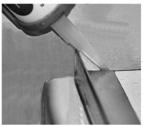
Step 13: Place one Side Jamb between the Bottom Track and the Wall into the wet Silicone. Find the center slot in the center of the side jamb and install a #8x1-1/2" (item#7) screw into the molly. <u>Use caution not to move the Bottom Track.</u> The side Jamb should line up with the pencil marks that you drew. When almost tight, take your level and check that the Side Jamb is plumb. If it is Plumb; then tighten the screw. Repeat Step 13 for the other Side Jamb.
