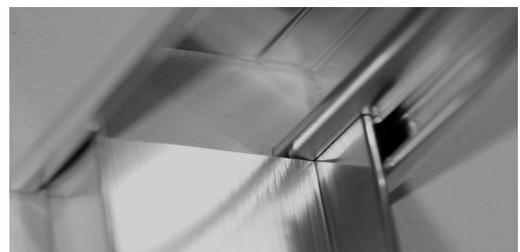
Step 21: On the inside face of the Header, Drill (1) 1/8" hole to the dimensions shown to secure the header to the Side Jambs. One hole on each end of the header. Use a Hand Screw Driver to install the #8x1/2" screw
