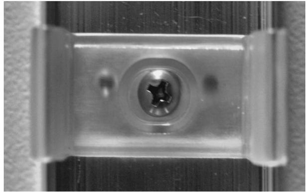
Step 16: Check the Side Jamb with the Level again and make sure it is still plumb. If it is; install the upper and lower bumpers. Recheck with Level again making sure the Side Jamb is still Plumb.
